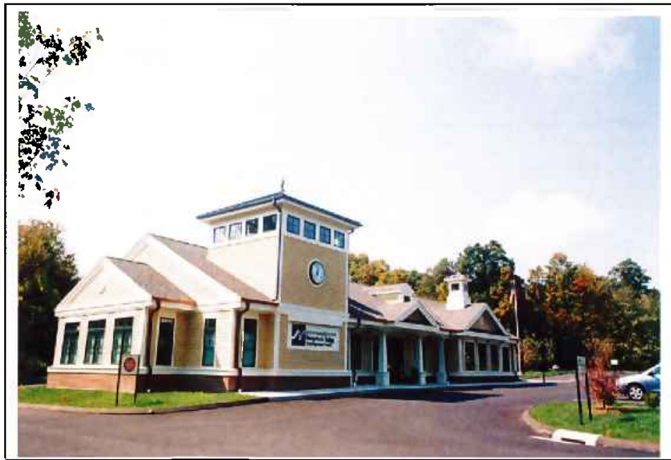
New commercial construction at 1570 Southford Road.
